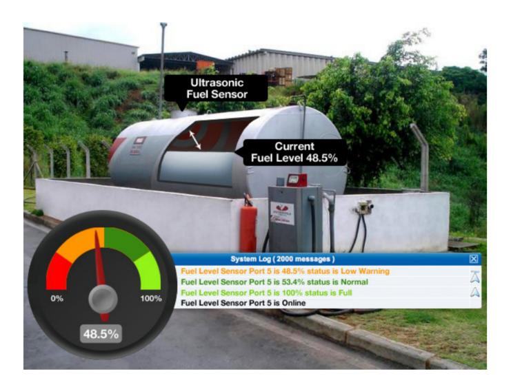
transmitted directly via Ethernet or an EDGE/GPRS/GSM Modem to the AKCess Pro Server. Sudden changes in Liquid Level or Liquid Volume can be used to trigger Notifications and Alerts to protect against theft and general Service Outages.
